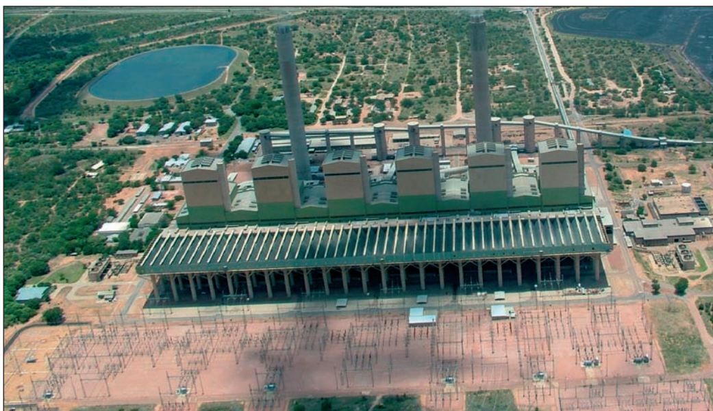
Figure 5: Aerial view of the Matimba Power Plant showing the ACC at the front of the power plant.
