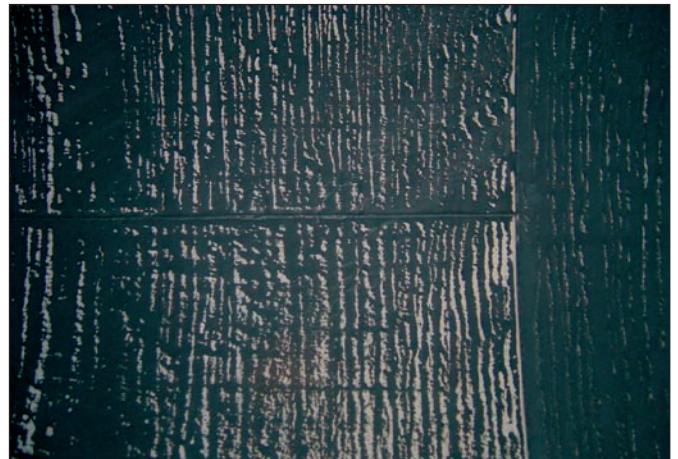
Figure 13: Minor bare metal (white) areas on black background as observed in the duct section H1 (see Figure 6 ). DHACI B.
