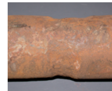
Backpass economizer tube with wall loss due to acid dewpoint corrosion.
