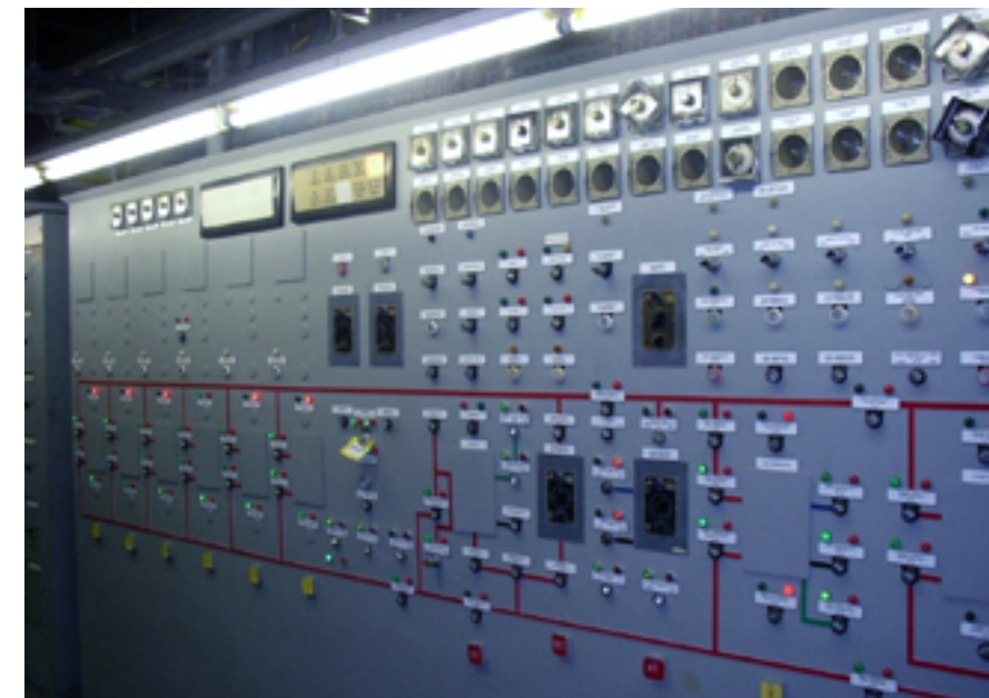
FIGURE 1. Condensate Demineralizer Panel at a BWR (Front Panel Face)
