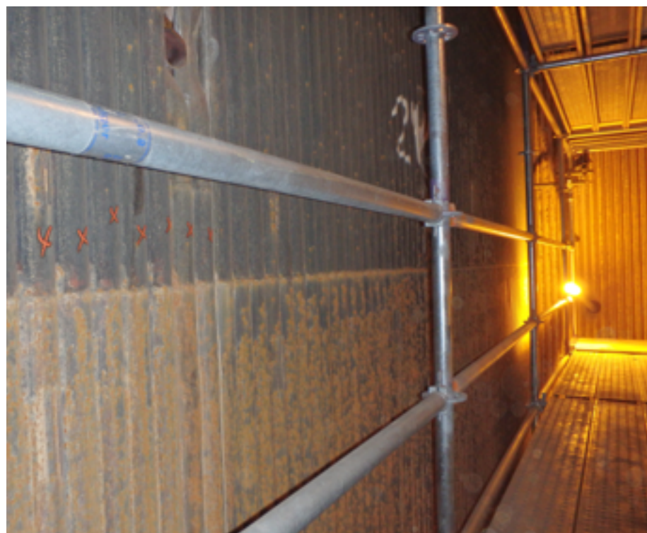
Thin edged rupture due to fire side corrosion
