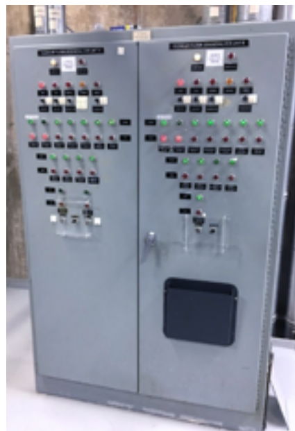
FIGURE 3. Original RWCU F/D Control Panel at James A. FitzPatrick NPP
