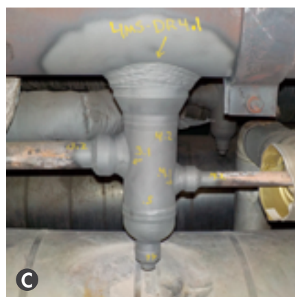
FIGURE 1. Examples of Proper Surface Prep Obtained by Grit Blasting at (A) a Saddle Weld, (B) a Tee with Multiple Welds, (C) Fillet Welds at Fittings, and (D) a Seam Welded Component
