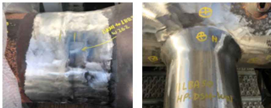
FIGURE 2. Examples of Good Surface Prep Obtained by Hand Grinding
