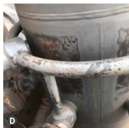
FIGURE 1. Examples of Proper Surface Prep Obtained by Grit Blasting at (A) a Saddle Weld, (B) a Tee with Multiple Welds, (C) Fillet Welds at Fittings, and (D) a Seam Welded Component
