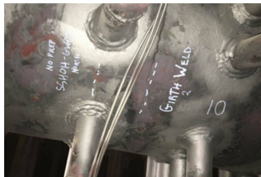
FIGURE 7. ABOVE AND BELOW Examples of Good Surface Prep Obtained by Grit Blasting at Header Stub Tube Welds (Note in the UPPER Image that a Header Girth Weld was Not Prepped for Inspection)
