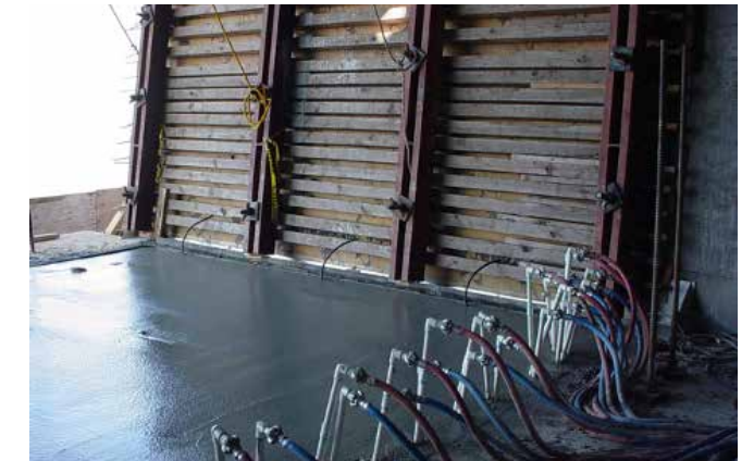
FIGURE 3. Concrete placement with active cooling to reduce concrete heat generation
