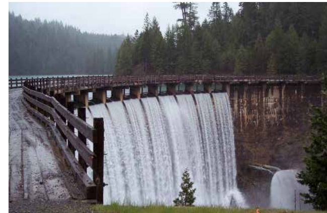
FIGURE 2. Concrete arch dam circa 1909, aging degradation Issues subject to increased flood and seismic demands
