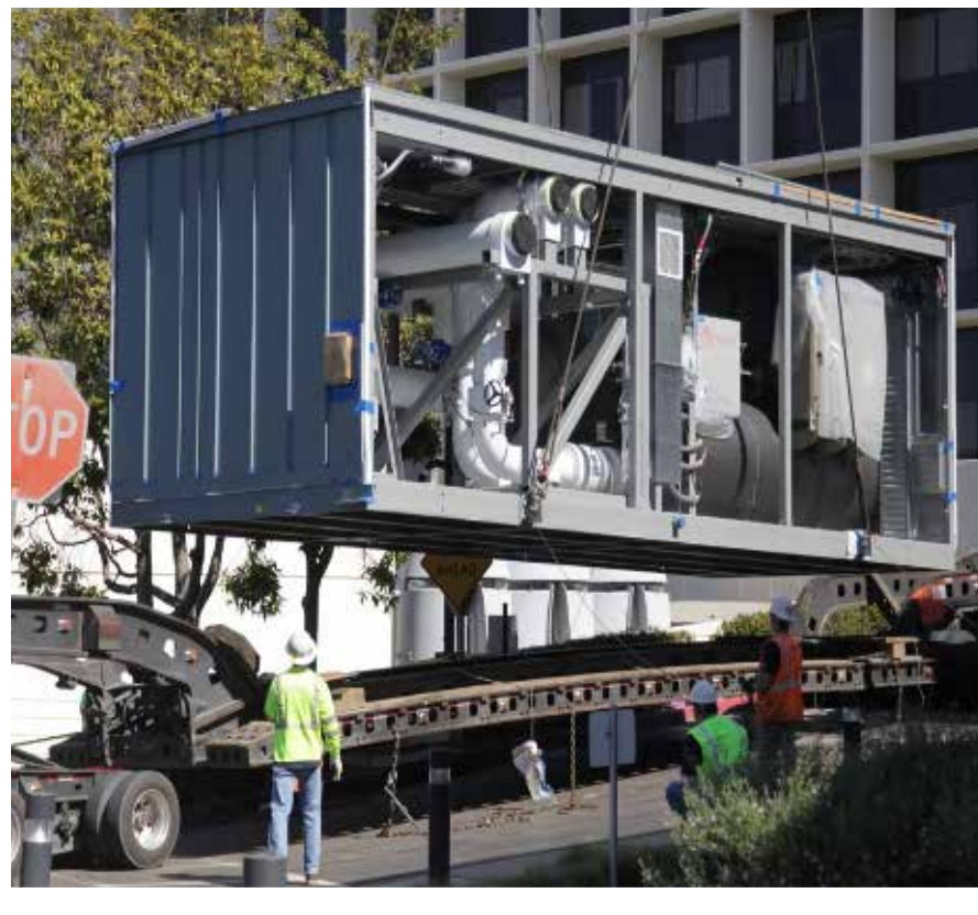
FIGURE 1. Lifting of Modular Central utility plant at Scripps Green Hospital, San Diego, California
