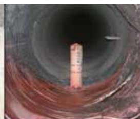
Cracked Liner
