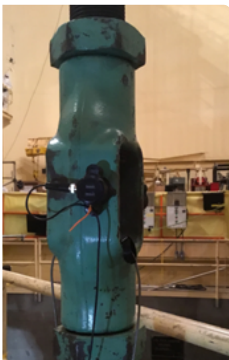
FIGURE 3. Close-up of AE sensor.
