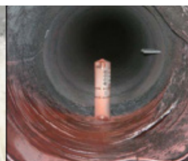
Cracked Liner
