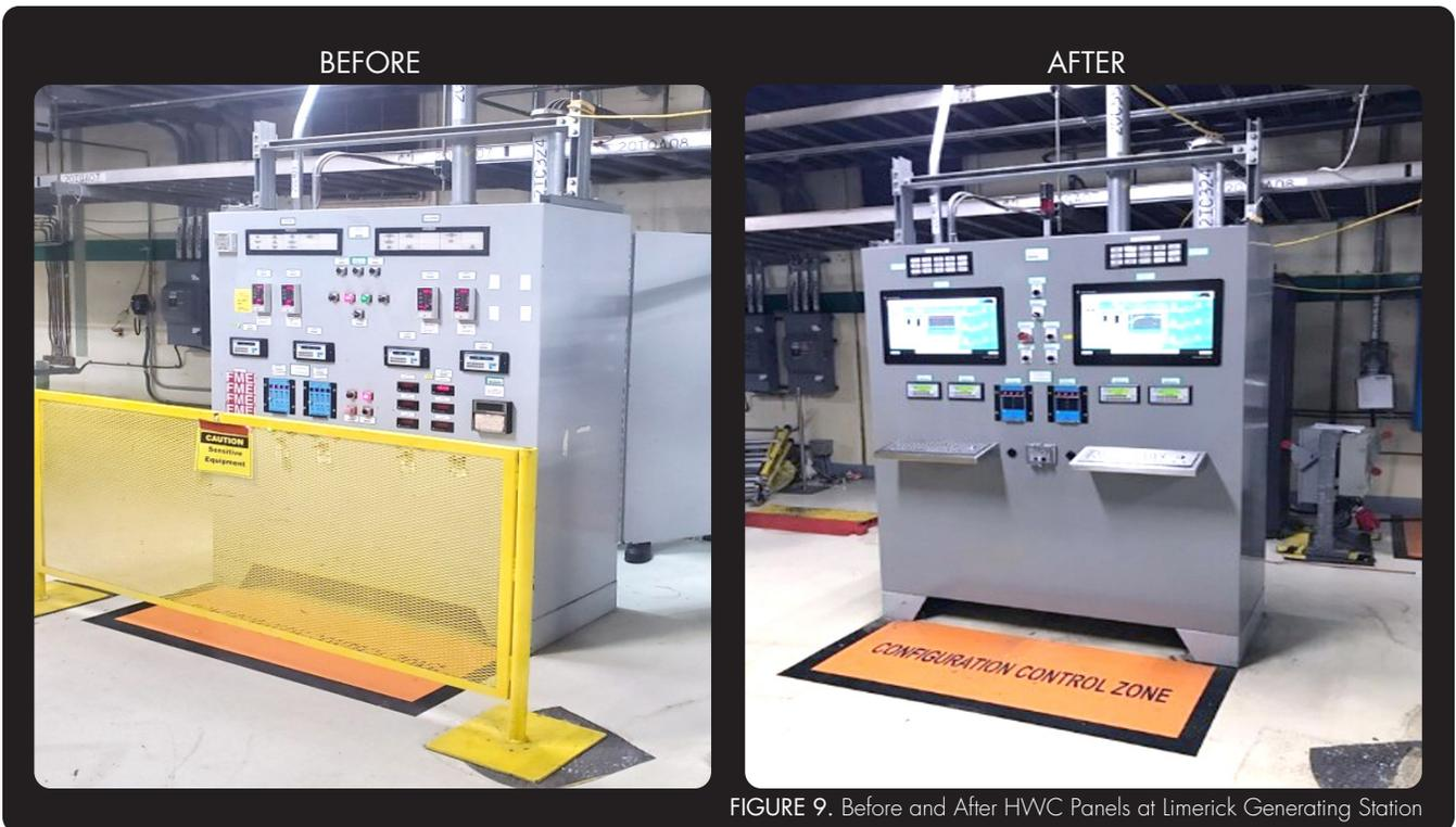
FIGURE 9. Before and After HWC Panels at Limerick Generating Station
