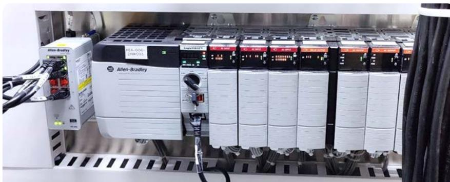
FIGURE 2. Allen-Bradley PLC (ControlLogix Platform)
