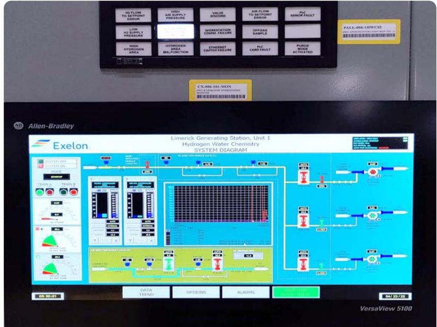
FIGURE 8. Limerick Unit 1 HWC Control System – HMI and O/I
