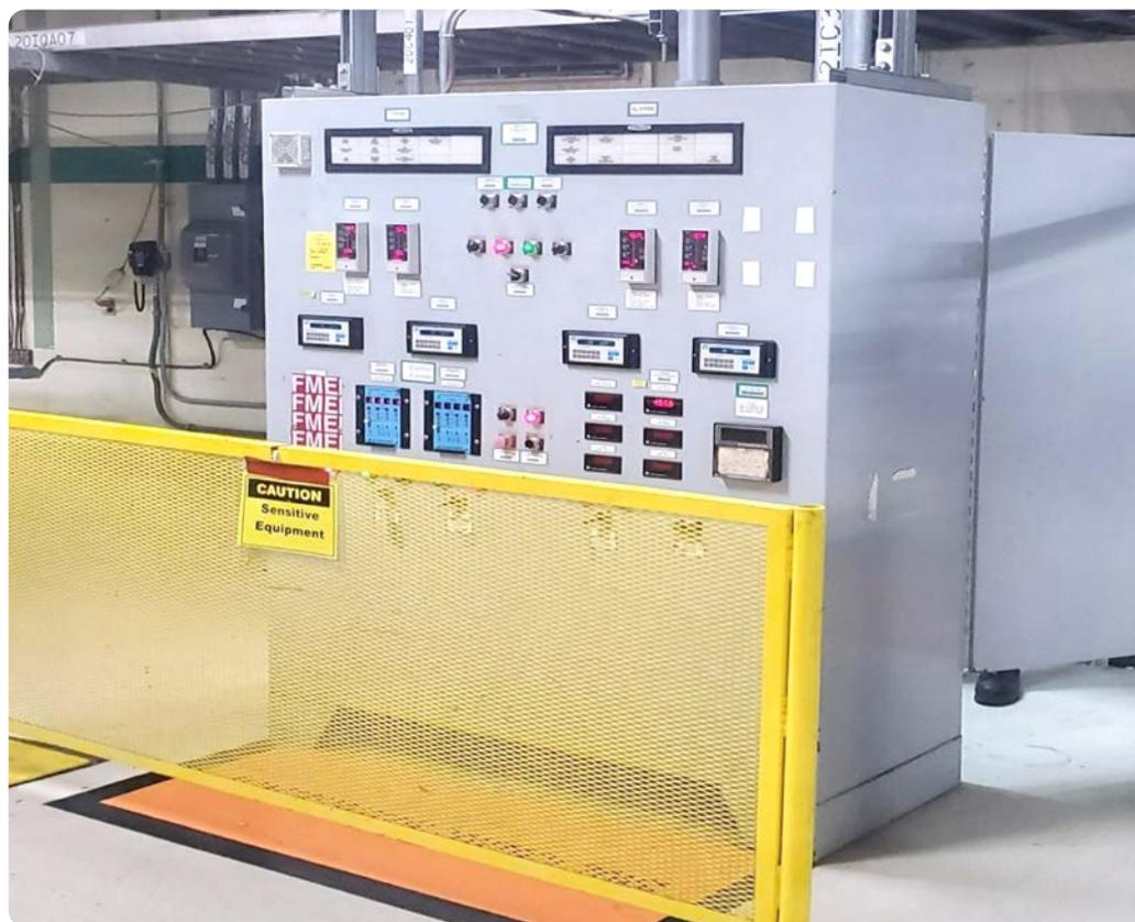
FIGURE 1. Previously Installed HWC Panel at Limerick Unit 2 (Front Panel Face)
