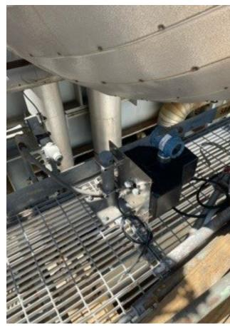
FIGURE 2. Winterization Package for Drum Level Transmitter
