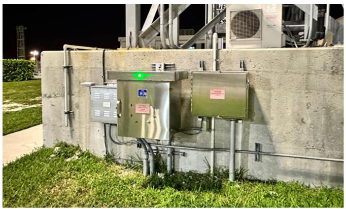
FIGURE 3. Rectifier Operating in Plant Protected Area
