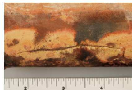
FIGURE 2. Longitudinal SCC in a stainless steel low-temperature superheater tube
