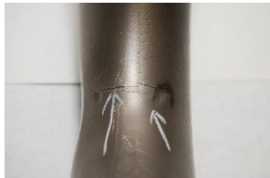
FIGURE 1. Circumferential stress corrosion cracking (SCC) in a stainless steel reheat tube on the OD (left) and ID (right)
