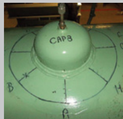
Figure 2. Typical encapsulation repair
