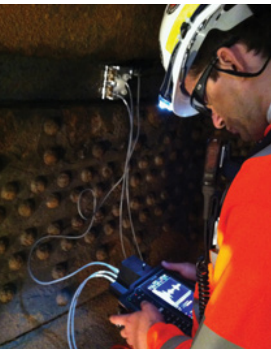
Figure 2. Inspection of the SAB1 penstock longitudinal lap joint showing the EMAT probe connected to the handheld electronics.
