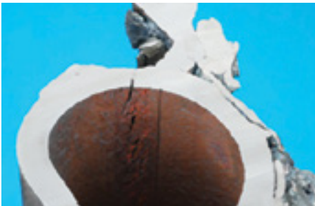
Figure 2. Cross-sectional views of the cracking shown in Figure 1. The parallel array of cracks is typical of corrosion fatigue.
