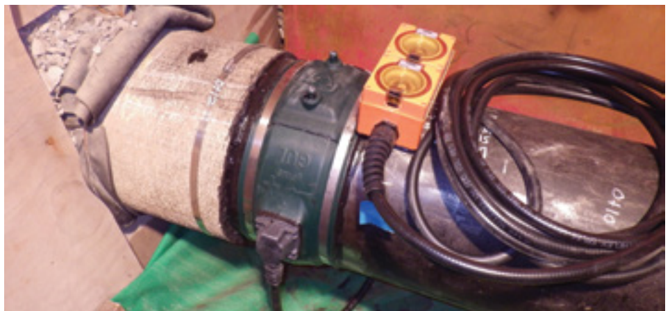
Figure 1. Photograph of a gPIMS™ transducer collar, manufactured by Guided Ultrasonics, Ltd. (GUL), permanently installed on a pipe inside an excavation.
