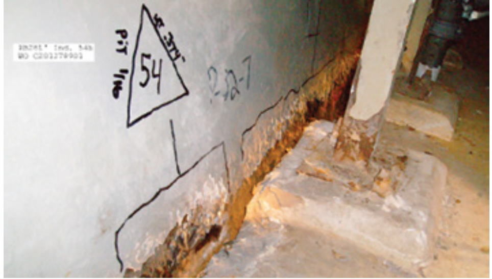
Corrosion at Carbon Steel Containment Liner-Concrete Floor Interface
