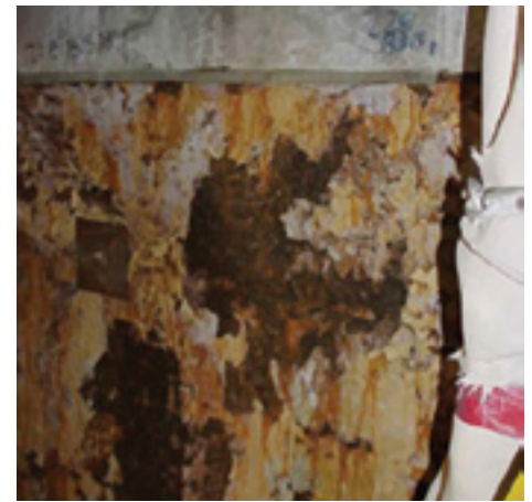
Corrosion at Carbon Steel Containment Liner-Concrete Floor Interface and Top of Lowest Liner Panel
