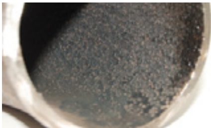
FAC damage in an LP Evaporator Elbow
