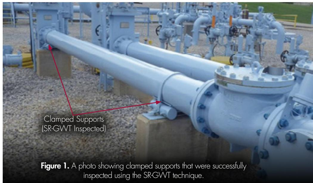
**Figure 1.** A photo showing clamped supports that were successfully inspected using the SR-GWT technique.
