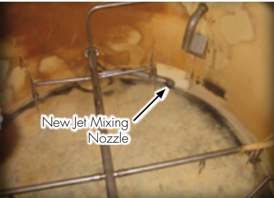
**Figure 3.** Phase Separator Tank Modification (BWR 4)
