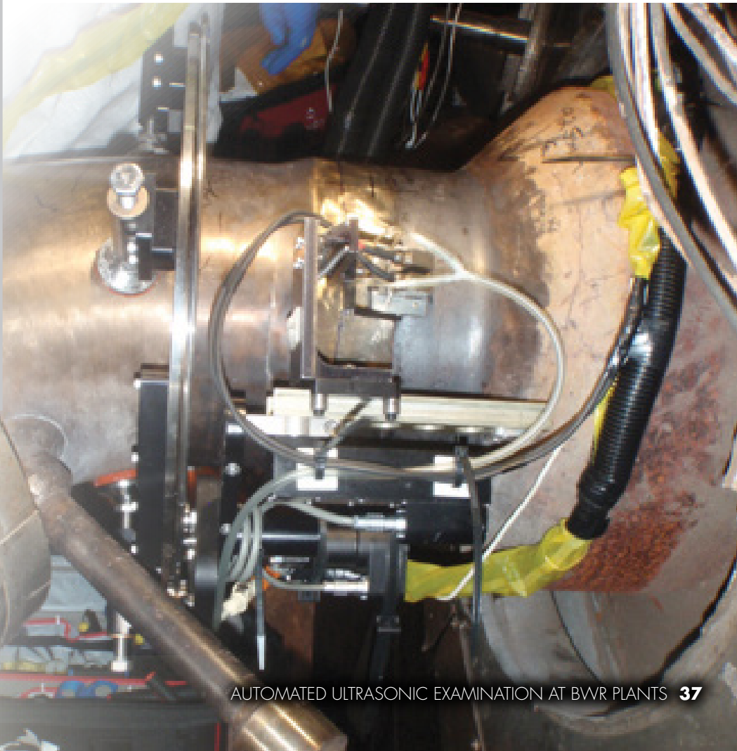
Structural Integrity's custom designed and in-house fabricated scanning system is shown mounted on an N5 Nozzle-to-Safe End DM weld
