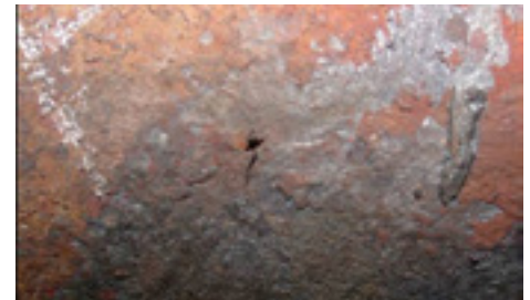
Figure 1. Pinhole leak on OD surface of waterwall tube
