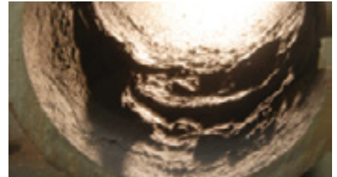
Heavy deposits on ID surface
