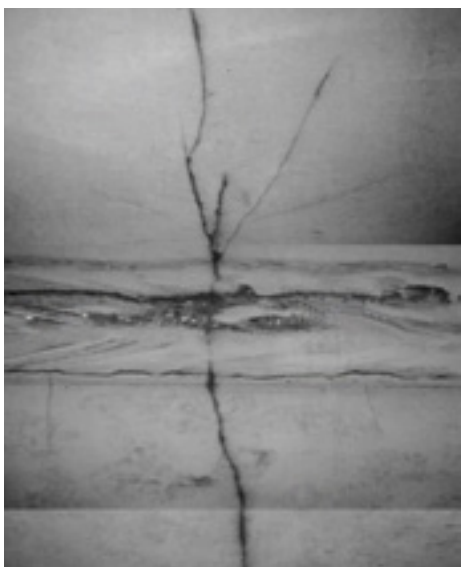
Photograph illustrating atypical cracking observed in domestic BWR core shroud.
