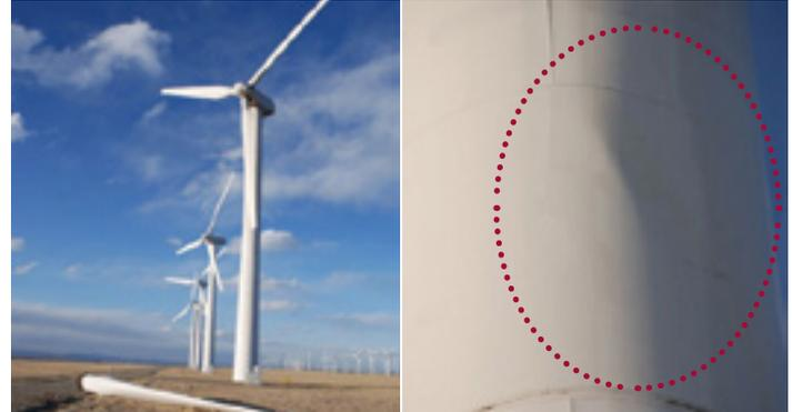
**Figure 1.** Site inspection for fractured blade and impacted tower.
