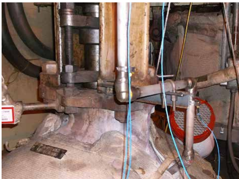
FIGURE 3. Smallbore Line Post-Repair Monitoring
