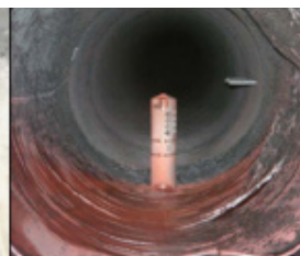
Cracked Liner
