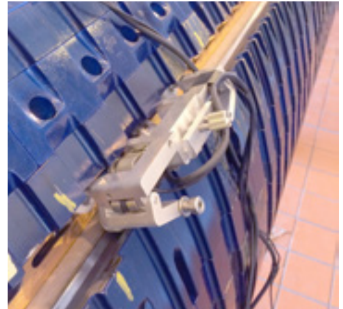
Generator rotor dovetail inspection
