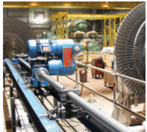
Rotor bore machining and surface conditioning
